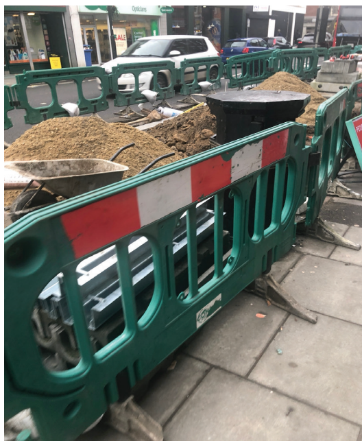
Work has started again on High Street
