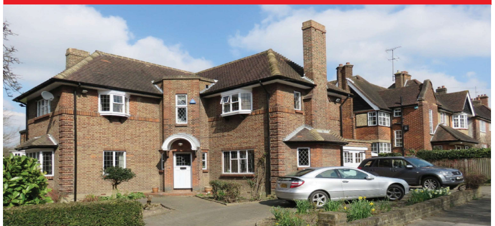
No.1 Sunset View, a fine Arts & Craft house has been nominated for the Local List. Extensions to the side and back of the property have been refused
